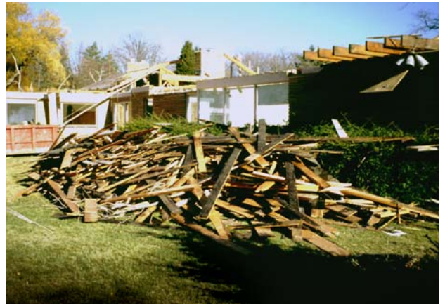
Valuable lumber being salvaged for reuse.
