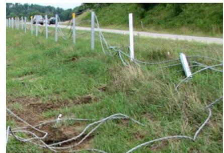
After an impact, the system will require some repair. Under most impacts, the HTCB will still maintain its original cable height and may be able to withstand additional hits. Even with this capability, it is recommended that the system be repaired as soon as possible. Because of the ease of repair, repairs can usually be done in a short period of time.
