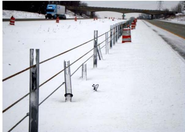
During the road patrol, pay particular attention to the end terminal post and the connection between the cable(s) and the cable terminal foundation. It is imperative that each cable be properly attached to the cable terminal foundation. Disconnected cables, improperly connected cables, and damaged end terminal may seriously compromise the functional ability of the system. These types of repairs may take additional time and may require re-tensioning of the entire run of cable.
