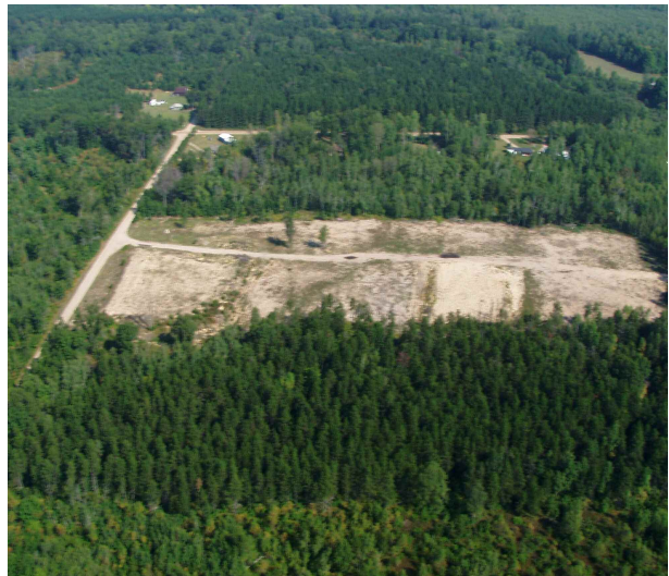
Aerial view of site after cleanup grant completed.
